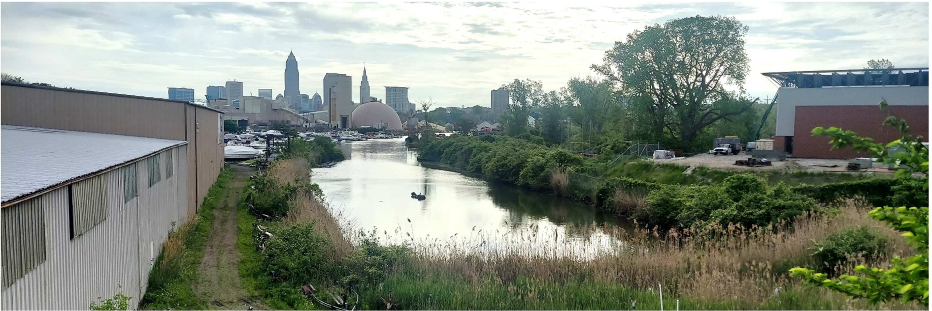
Figure 30: City owned, abandoned graving dry dock where Concepts G & H diverge from existing Shoreway alignment
