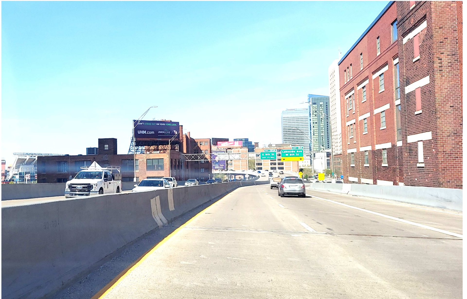
Figure 32: Photo of existing Shoreway in Warehouse District looking east
